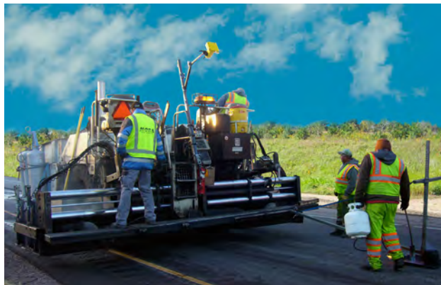
Figure 4: Paving machine controlled by the Big Sonic-Ski leveling system
